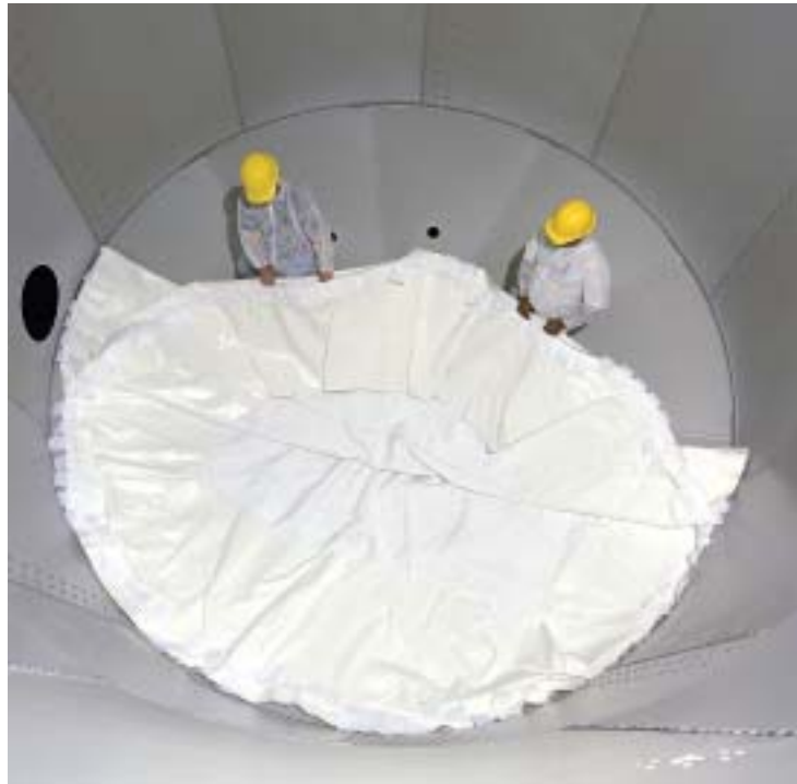
▲ Specially designed permeable fabric is laid over air manifold openings (hole between men) to help aerate flour and assure 100% flour discharge. SHICK
